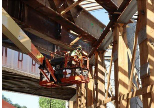
**Lone Hill Ave. Bridge (Glendora):** With the center columns and both abutments completed, crews are now focused on assembling and installing the falsework over Lone Hill Ave. The falsework is the temporary support for the super-structure as it is built across the street and is made up of a combination of steel and wood beams. Crews are currently assembling the parts for the falsework on-site (photos below). Once in place, the falsework will span from abutment to abutment.
