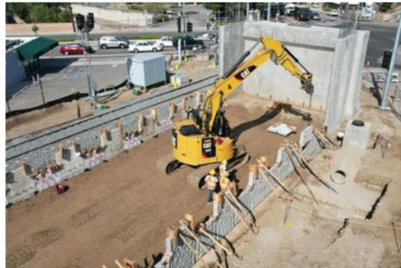
Across the intersection, the east approach for the bridge (photos above) continue to take shape as crews construct the retaining walls. The retaining walls for both approaches consist of custom form panels that feature the project's citrus design.
